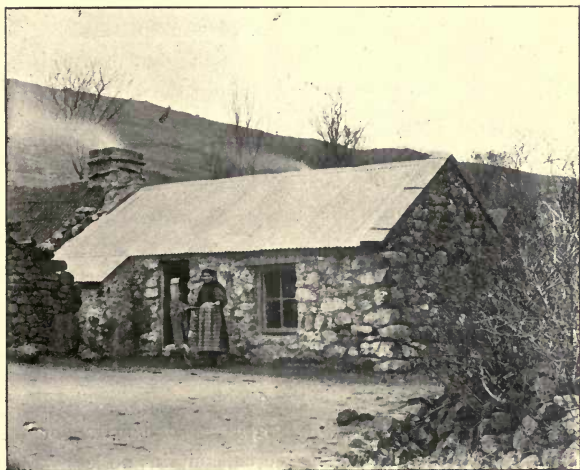
New-roofed (Corrugated Iron) Cabin and Spinning Wheel, Leenane. Notice also the Modern Window.
